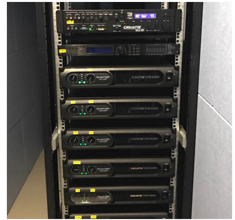
▲ Christie Vive Audio Class D amplifiers installed in one of the halls in MZC Quanjing Cinema.
