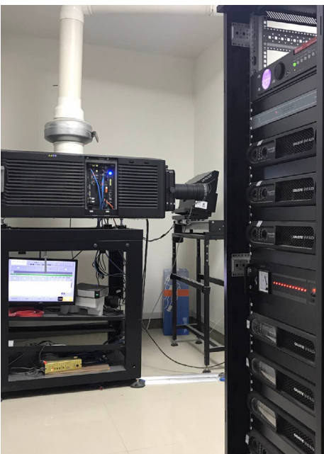
▲ The projection room of Hall 2 auditorium is fitted with a Christie CP2230 cinema projector, and Vive Audio Class D amplifiers.
