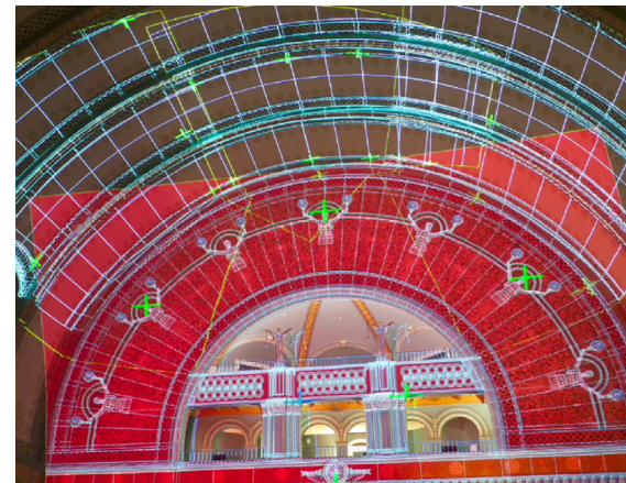
▲ Performing a laser scan of the end wall of the Grand Hall
